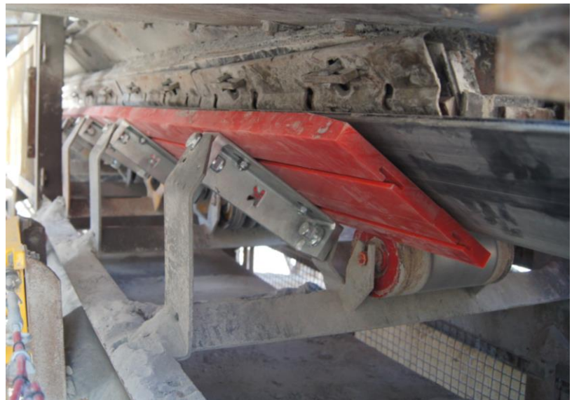
Right: images taken of K-Sure Belt Support after installation.
