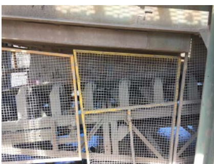
ABOVE Image of Transfer point BEFORE Conveyor Upgrade
