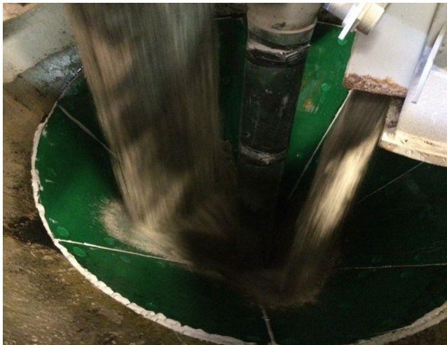
K-Superline® after installation at Dandenong, Sept 2014
