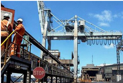
Photo on site of the Port Pirie bulk handling systems.
