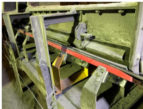
LEFT Image AFTER Installation
