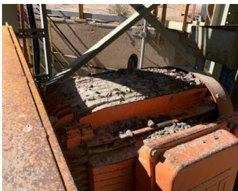
ABOVE Image BEFORE Installation
